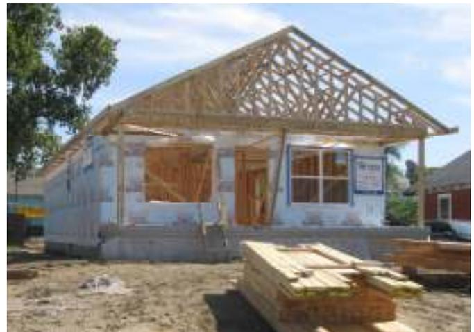
The roof trusses are in place, and some of the framing has begun on the inside of the house.
